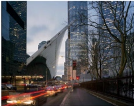
NORTH SIDE - SPRING STREET 2011
